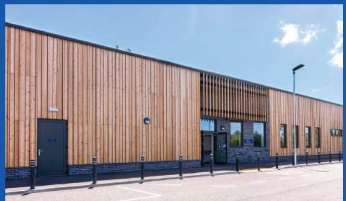
ISG - SFS, Timber cladding
