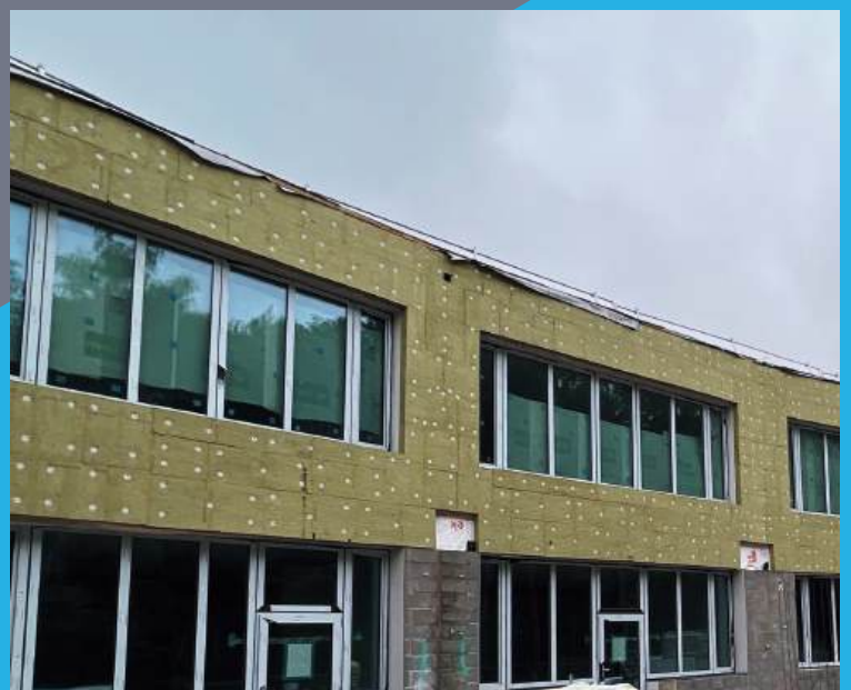
BAM - EWI, Render, Timber cladding
