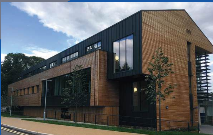
Willmott Dixon - SFS, Timber cladding
