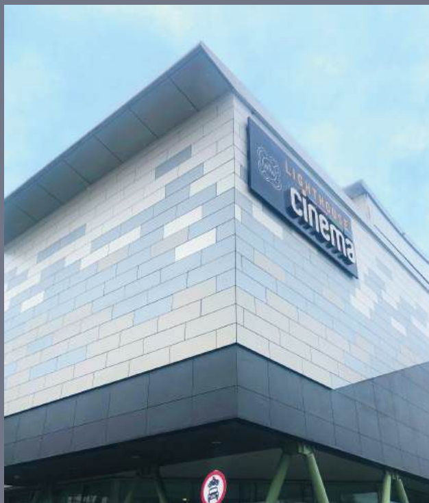
ISG - Rainscreen cladding
